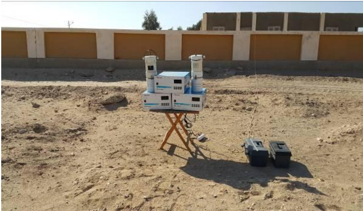
Figure 3-1 ambient air quality monitoring system
