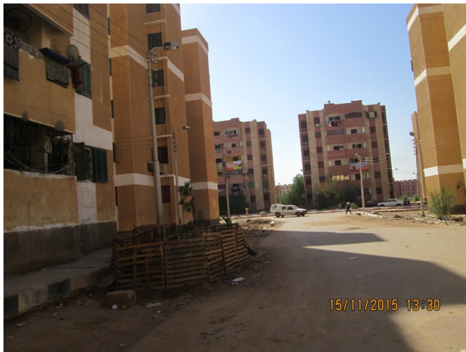
Figure 4-8: Local streets in Aswan city
