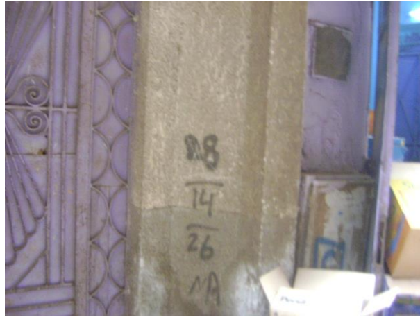
Figure 4-6: prevalent building type
