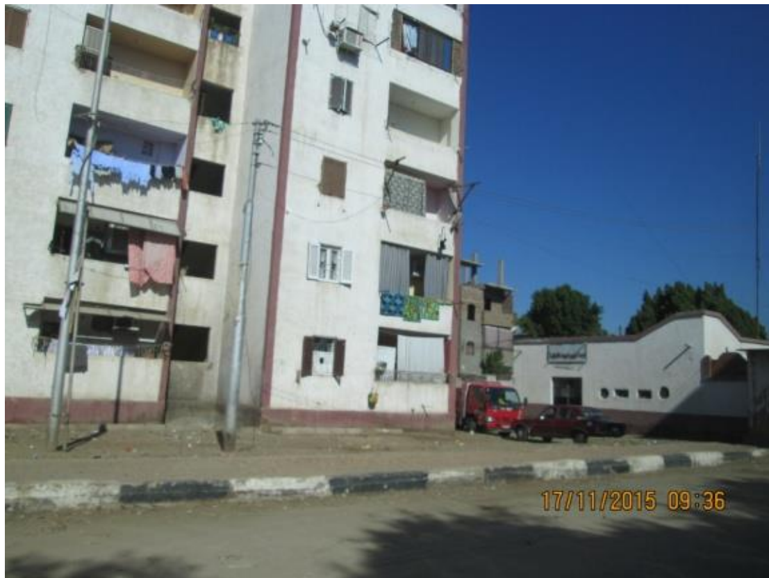
Figure 4-5: Residential building in Edfu city
