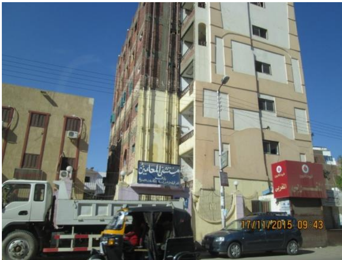
Figure 4-6: Newly constructed dwelling in Edfu city
