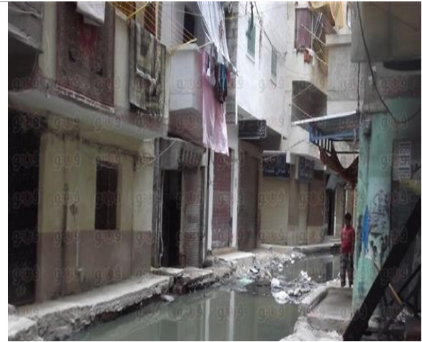
Figure 4-1: Buildings in Al Mandara
