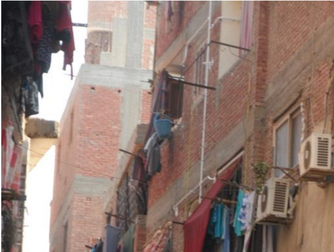
Figure 4-8: Typical red brick structures in El Khosous
