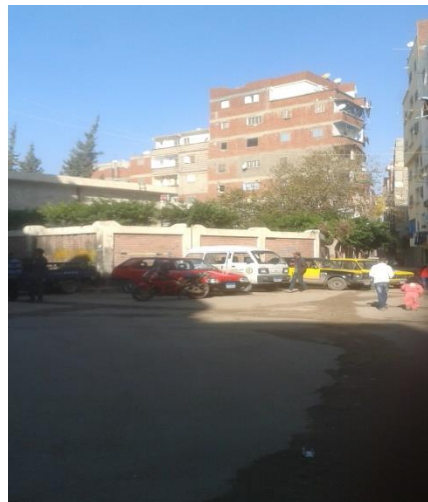
Figure 4-9: Buildings in Hagar El Nawateia
