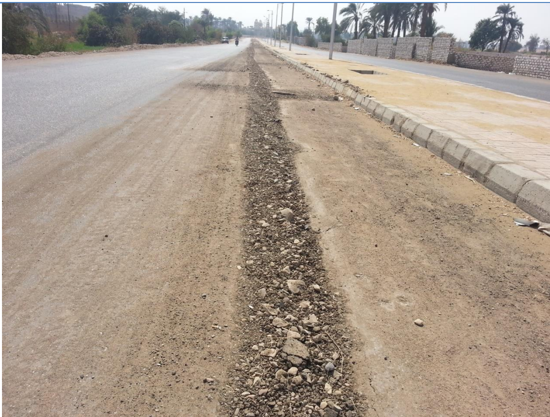
Figure 2-5: Digging the main roads close to the PRS in Qena
