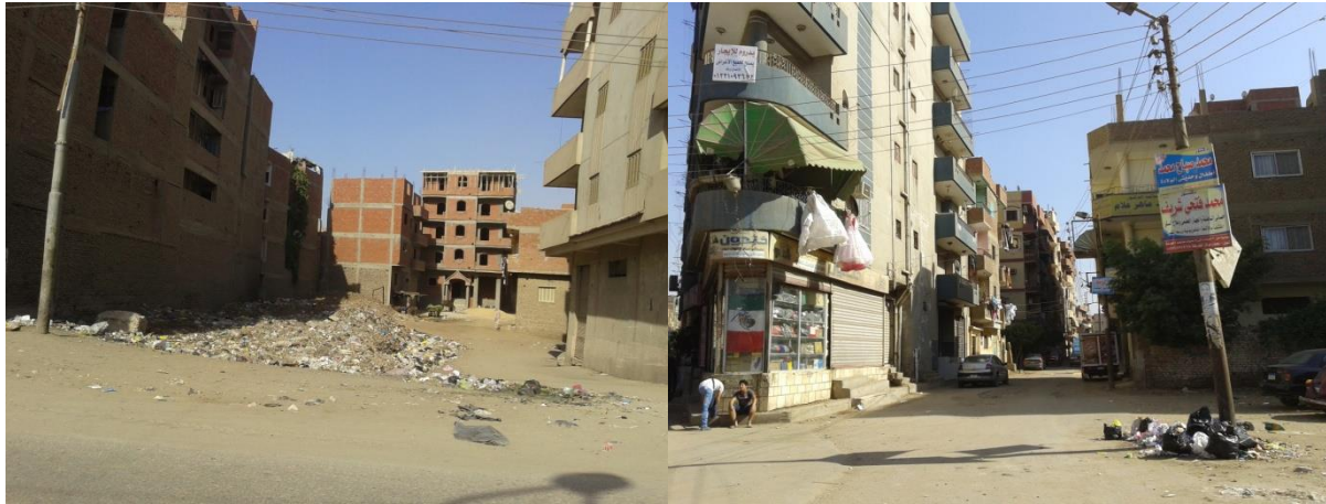
Figure 4-7: Newly constructed buildings
