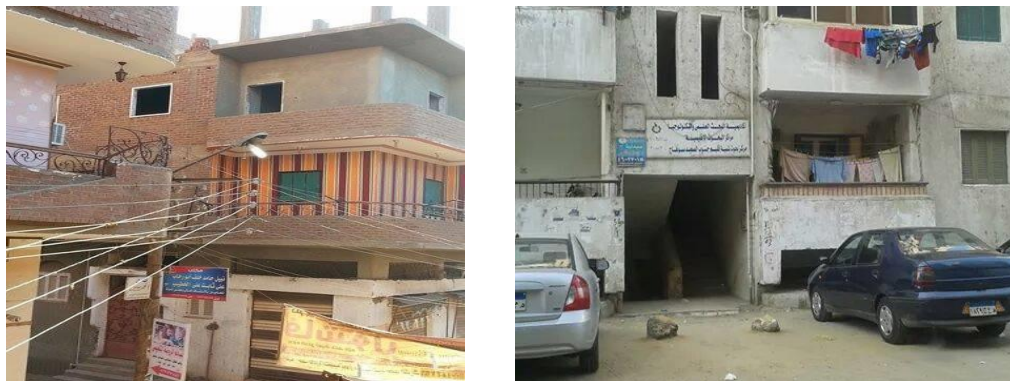
Figure 4-15: Newly constructed dwellings
