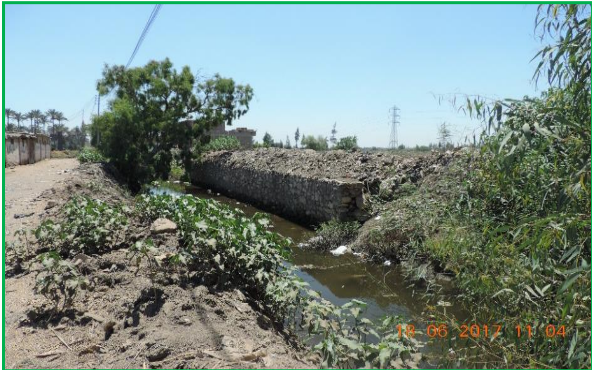
Figure 4-3: Shows small branch from EL-Jawwasiyyah canal in Belqas district.
