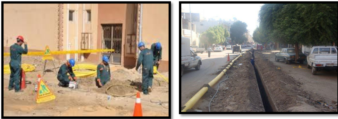
Figure 5-4: Open Cut by ReGas
