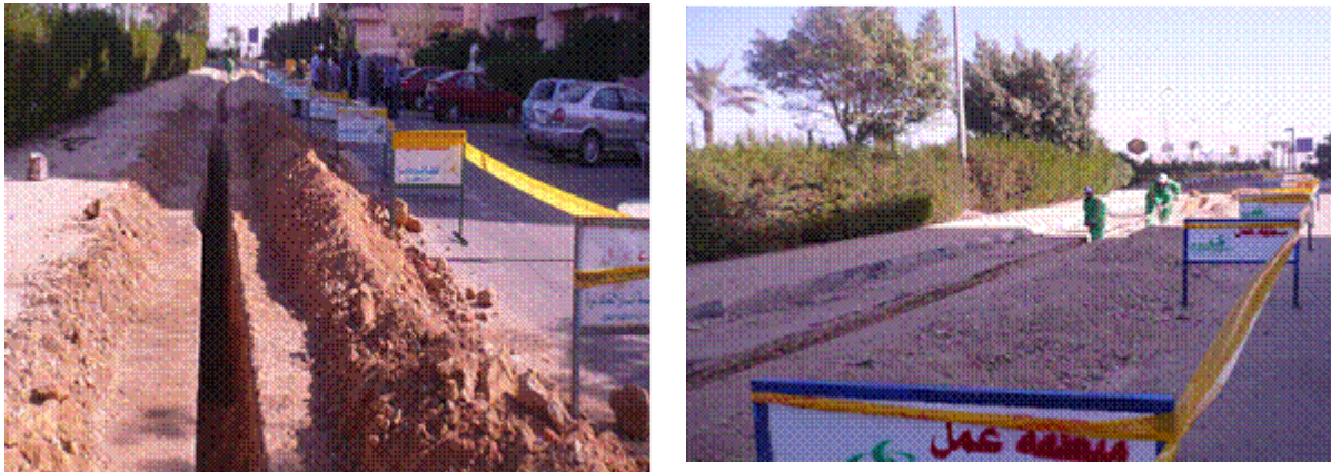
Figure 2-4: Example of an excavated trench prior to pipe laying.
