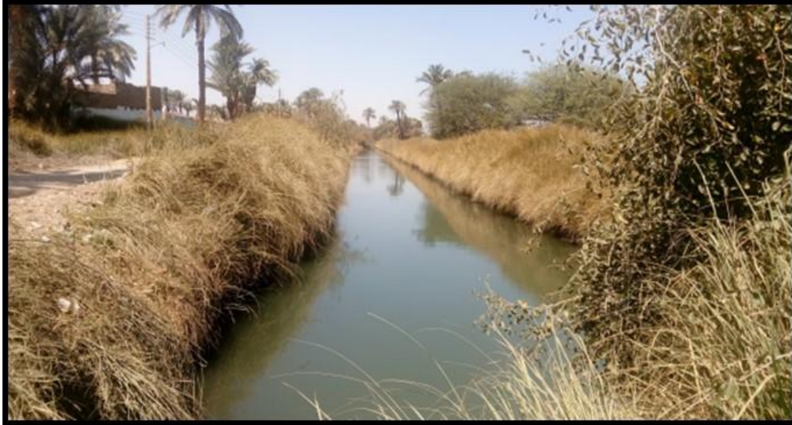
Figure 4-3: Canal of Kalabya
