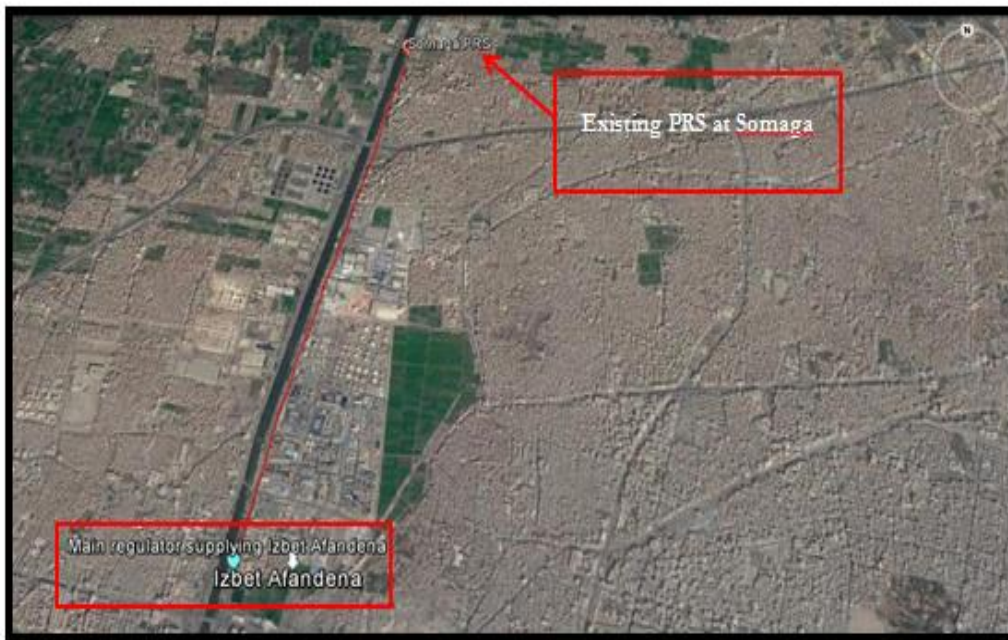
Figure 2-6: Main feeding line to Izbet Afandena
