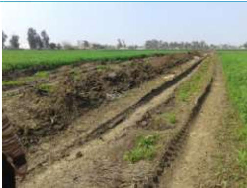
Figure 2-1: Damaged area of land in Kafr El Zayat route
