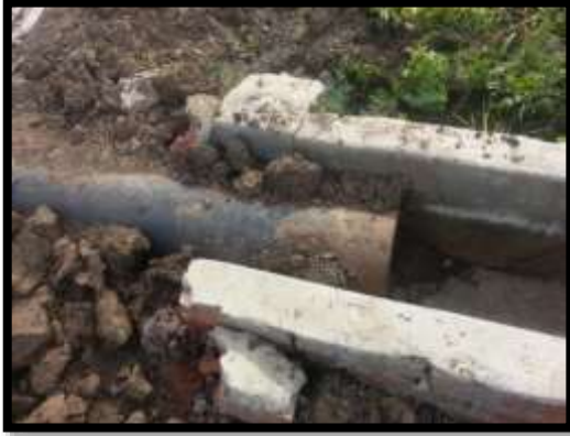
Figure 1-2: Irrigation channel in the route path
