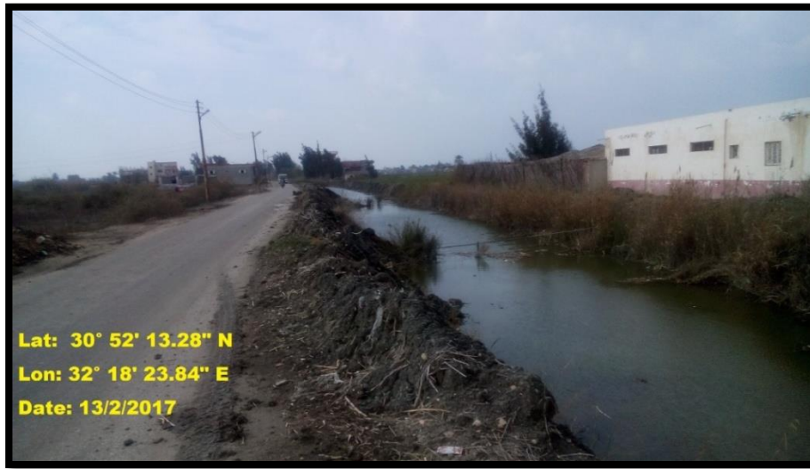
Figure 4-9 Drainage next to Port Said –Ismailia road and PRS Qantara Gharb
