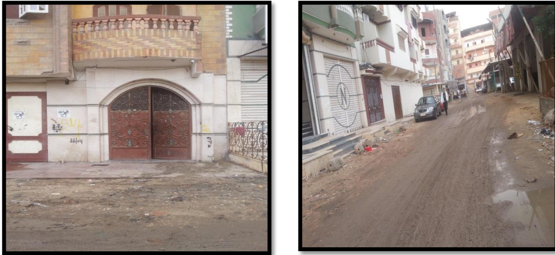
Figure 4-24 Street conditions in Qantra Gharb
