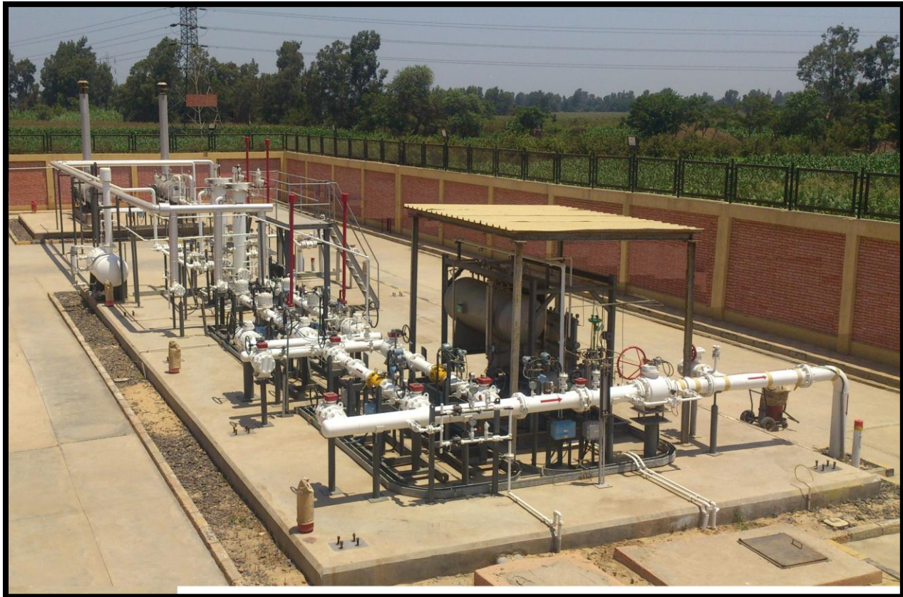
Figure 2-7: Typical example of the planned PRS”
