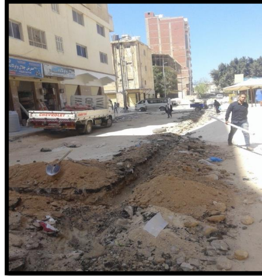
Figure 2-8 Typical trench for PE pipes
