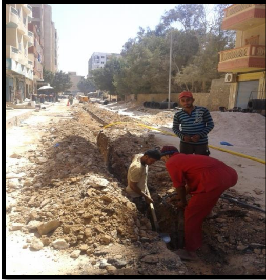
Figure 2-8 Typical trench for PE pipes
