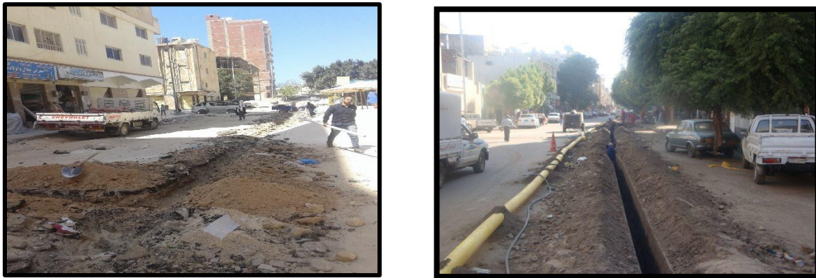
Figure 5-4: Open Cut by ReGas
