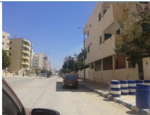
Figure 4-9 : Local street from El Galaa road
