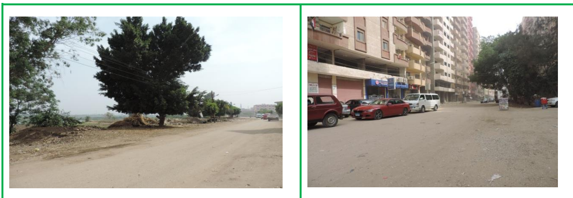
Figure 4-7: Pictures showing Streets Conditions at Kafr Shukr.
