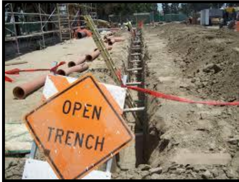
Figure 2-5 Open Trench Example
