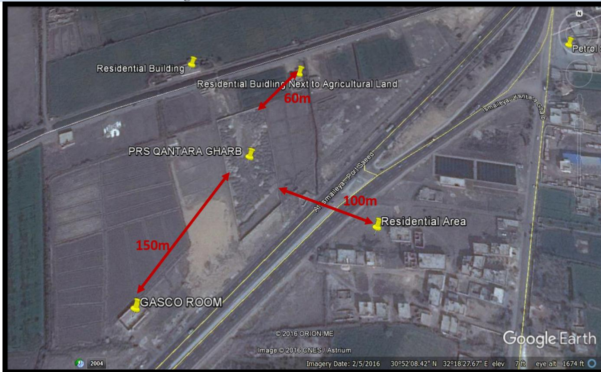
Figure 2-4 PRS Qantara Gharb and the surrounding area
