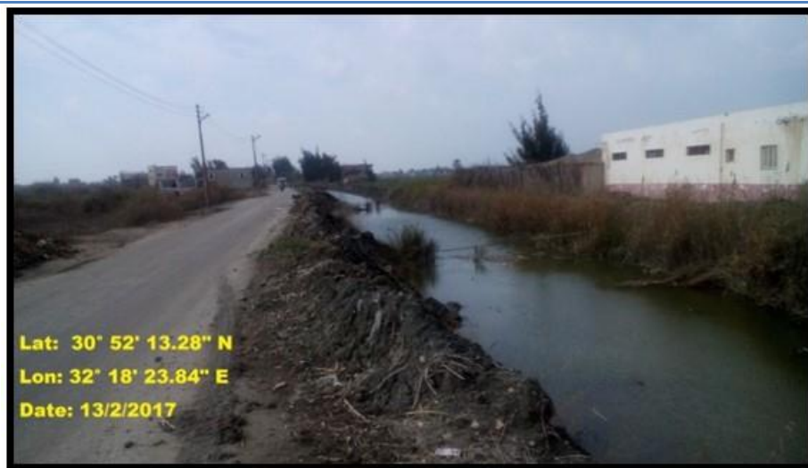
Figure 4-8 Drainage next to Port Said –Ismailia road and PRS Qantara Gharb
