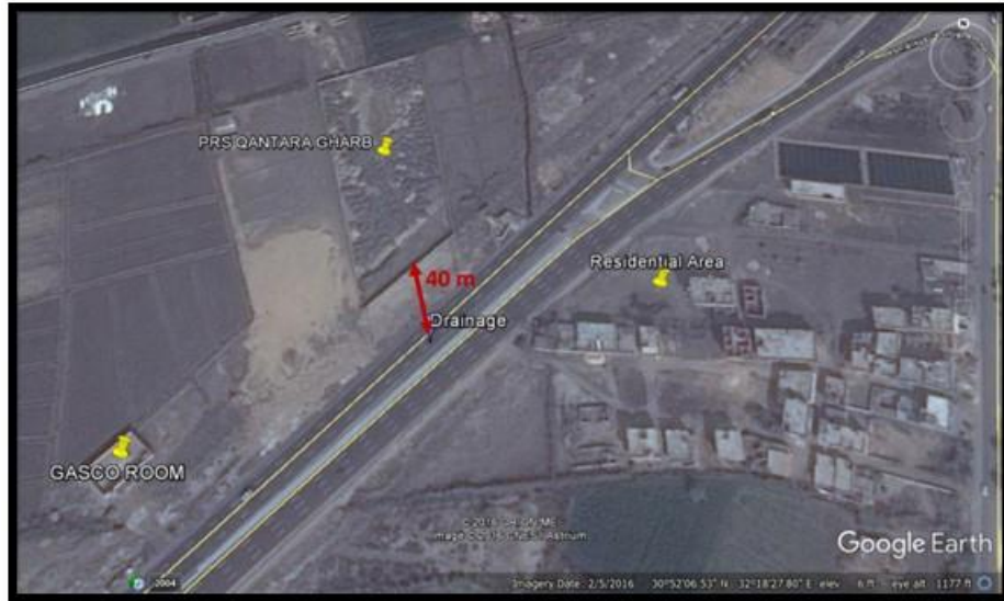
Figure 4-9 Drainage next to Qantara Gharb PRS
