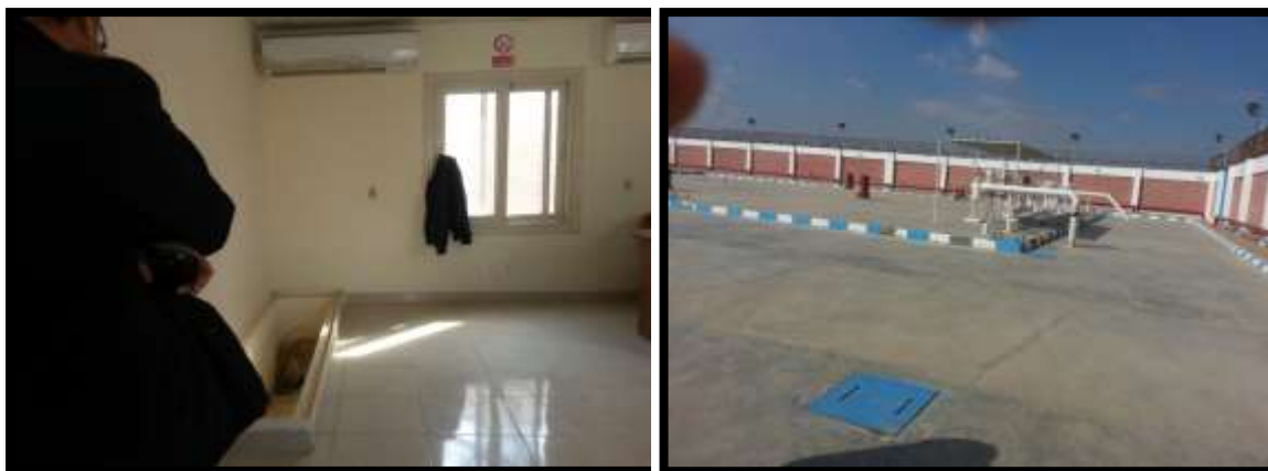
Figure 2-4: Control room in Qantra Shark PRS Figure 2-5: Qantra Shark PRS fence
