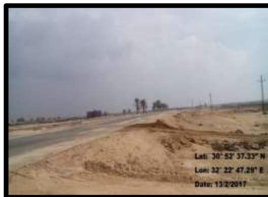
Figure 4-11: Ras Sedr- Qantra Shark Road adjacent to the PRS
