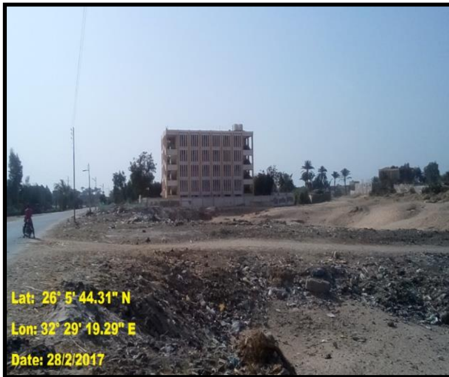
Figure 4-17 Ali Hassan school located close to the PRS site
