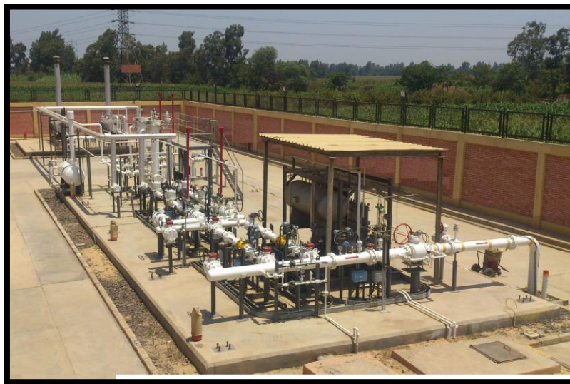
Figure 2-5: Typical example of the planned PRS
