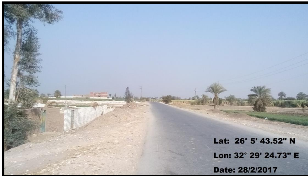
Figure 4-11: The road connecting El Marashda and Waqf city
