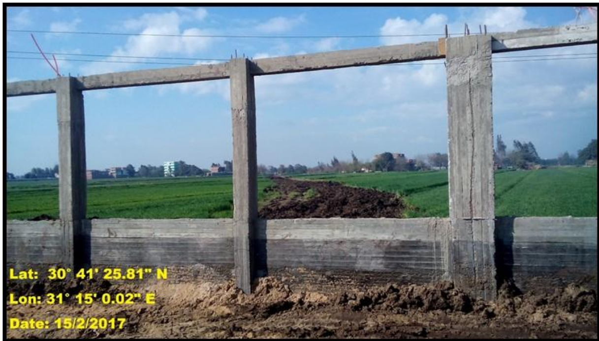
Figure 2-4: The route in front of the PRS
