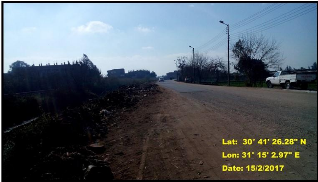
Figure 2-3: The road in front of the PRS
