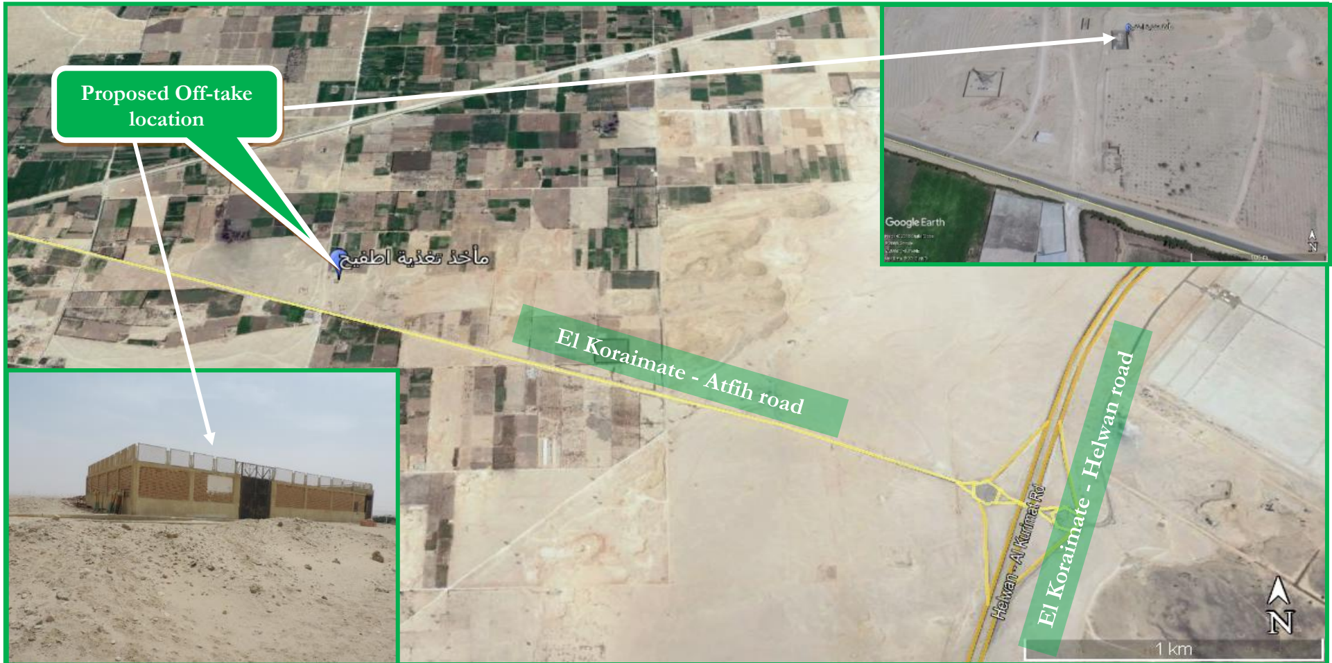
Figure 2-6: The proposed Location of the proposed Off-take point, which will be located inside Gasco valve room
