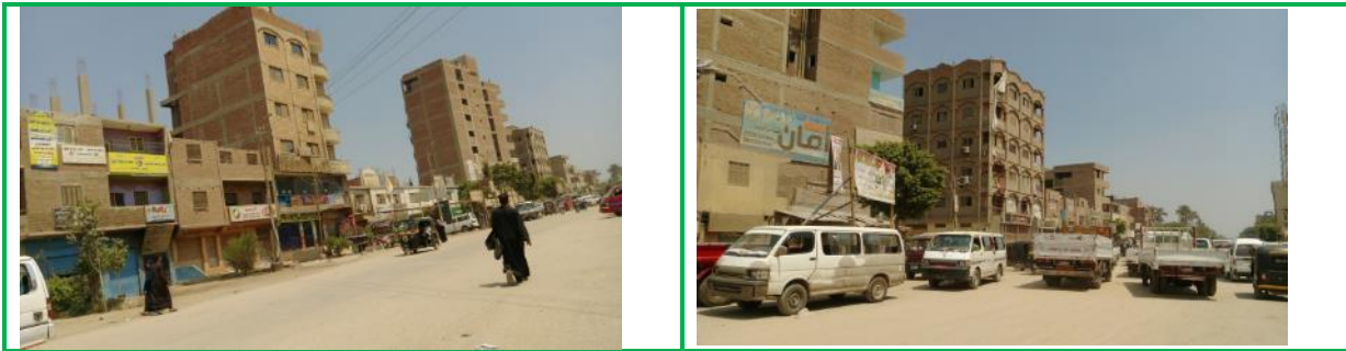
Figure 4-6: Pictures showing Buildings & Streets Condition in Atfih City
