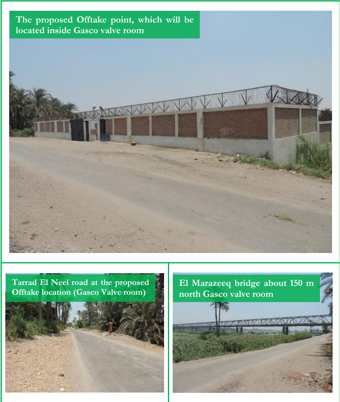
Figure 2-7: Pictures showing the proposed Location of the proposed Offtake point, which will be located inside Gasco valve room
