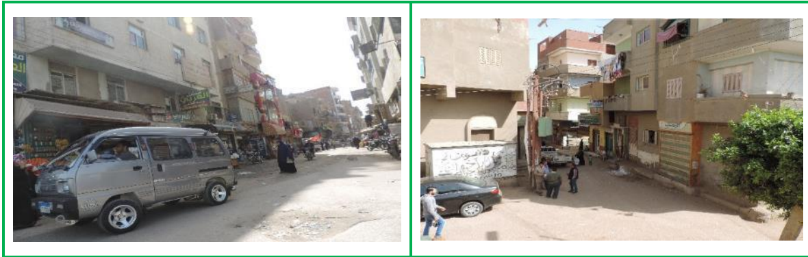
Figure 4-7: Pictures showing Building Condition at Ashmoon.
