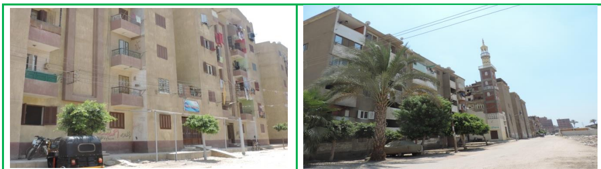
Figure 4-8: Pictures showing Building & Streets Condition in Qaha District.
