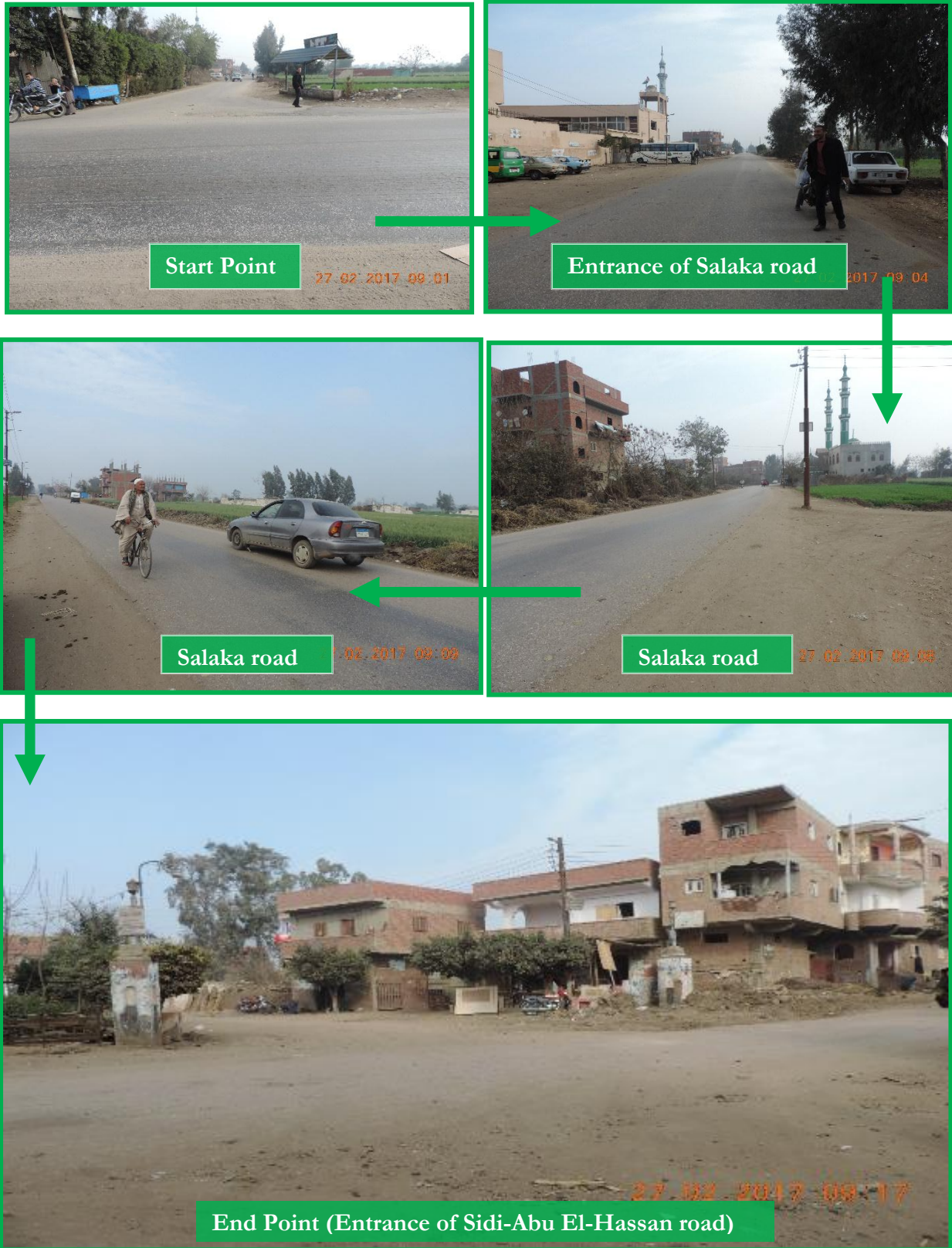
Figure 2-13: Pictures showing the proposed pipeline route feeding Salaka area
