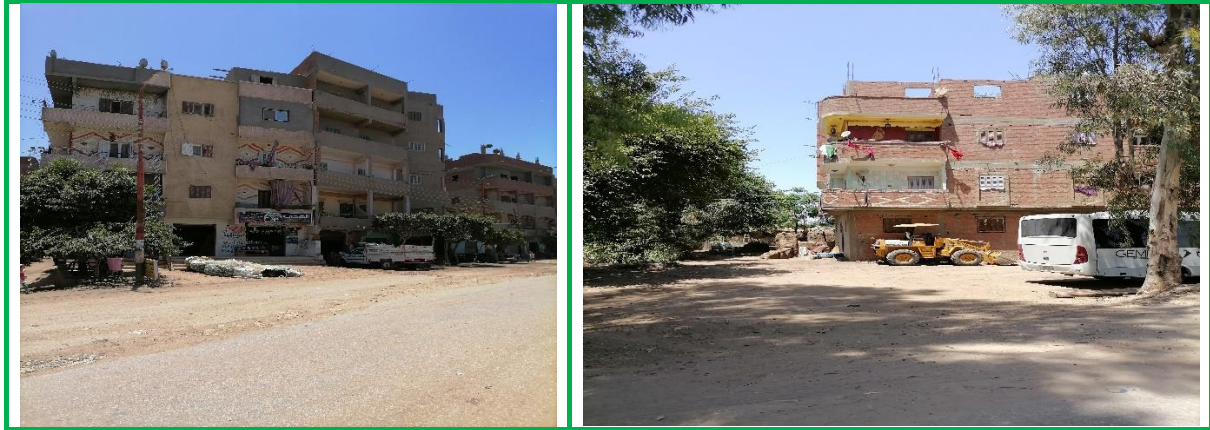
Figure 4-6: Pictures showing Building Condition at Shoubra bas.
