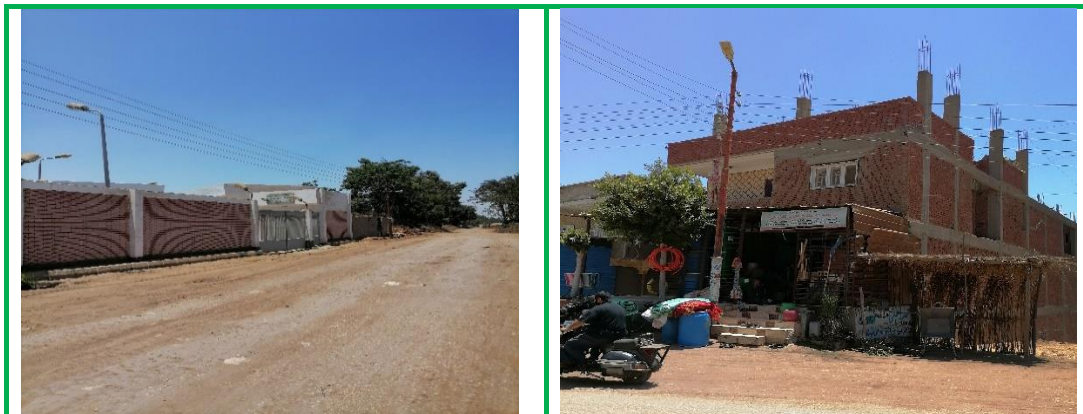
Figure 4-7: Pictures showing Streets Conditions at Shoubra bas.
