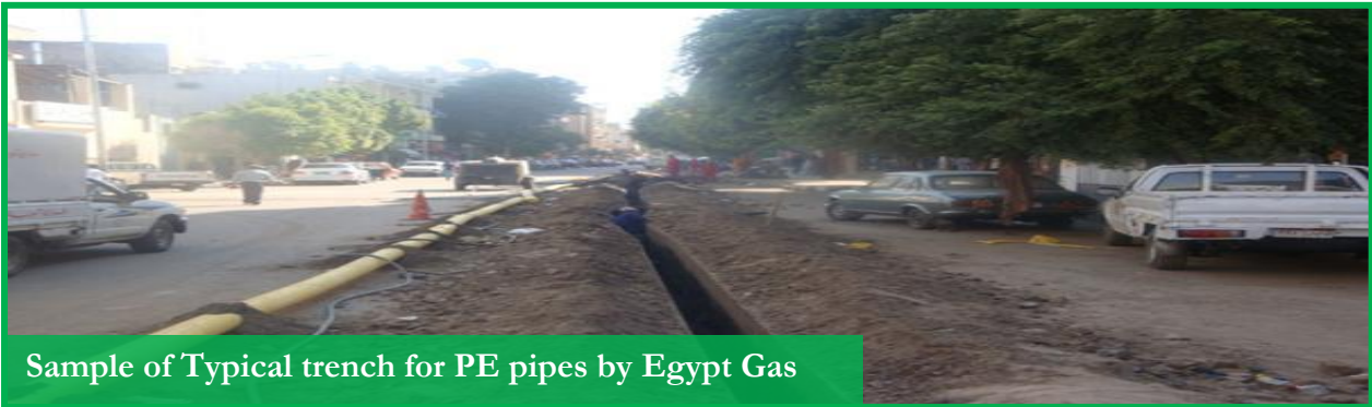
Figure 2-4: Picture showing sample of typical trench for PE pipes by Egypt Gas
