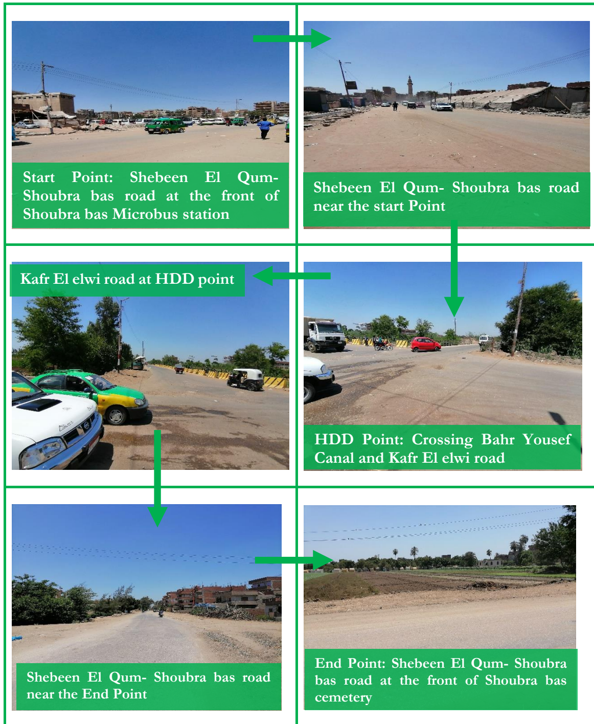
Figure 2-3: Pictures showing Shoubra bas intermediate pressure pipeline route.
