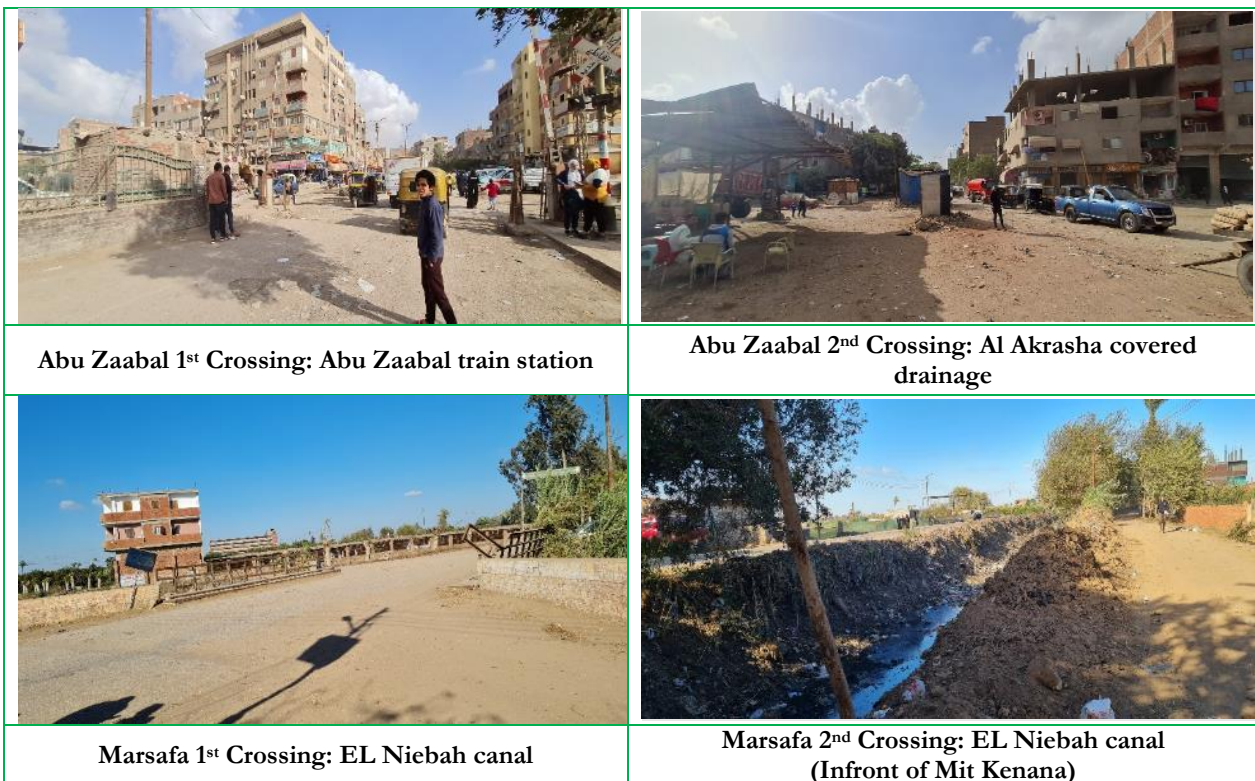
Figure 2-7: Pictures showing the proposed HDD crossings in Abu Zaabal and Marsafa districts
