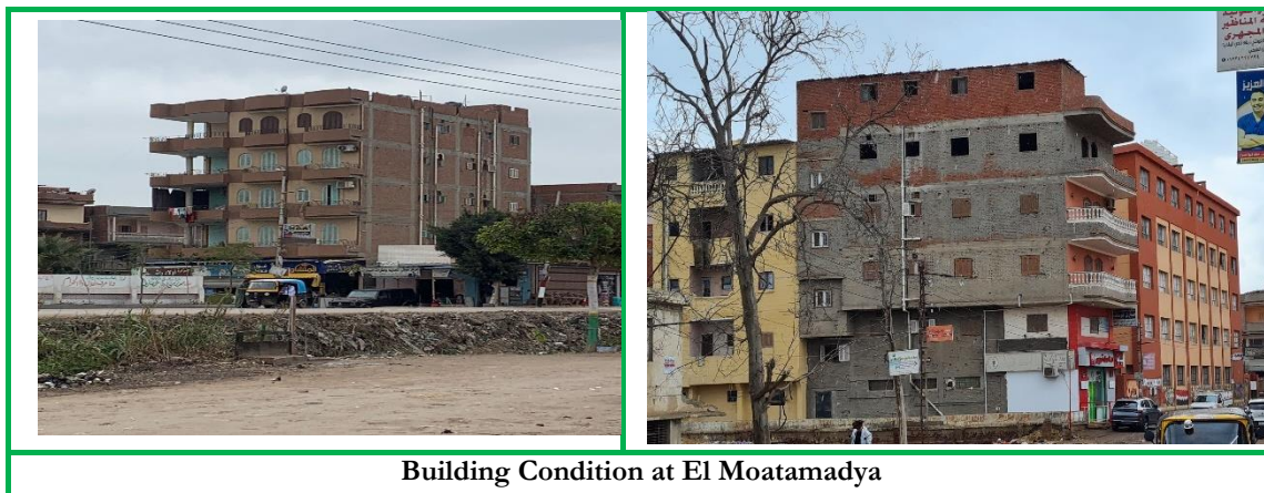
Figure 4-7: Pictures showing Building Condition at El Moatamadya.
