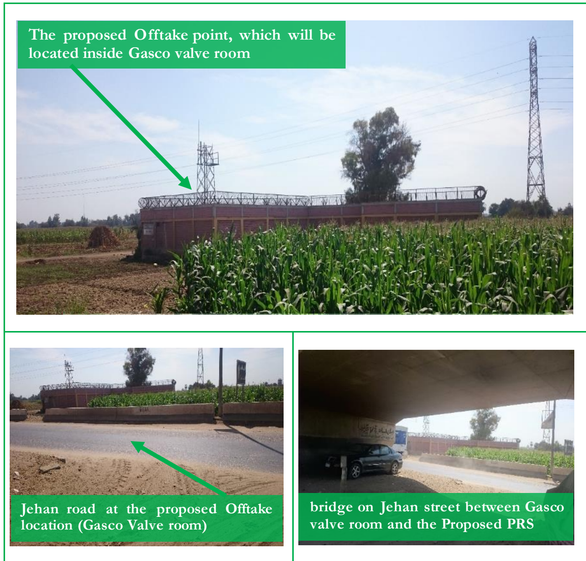
Figure 2-7: Pictures showing the proposed Location of the proposed Offtake point, which will be located inside Gasco valve room
