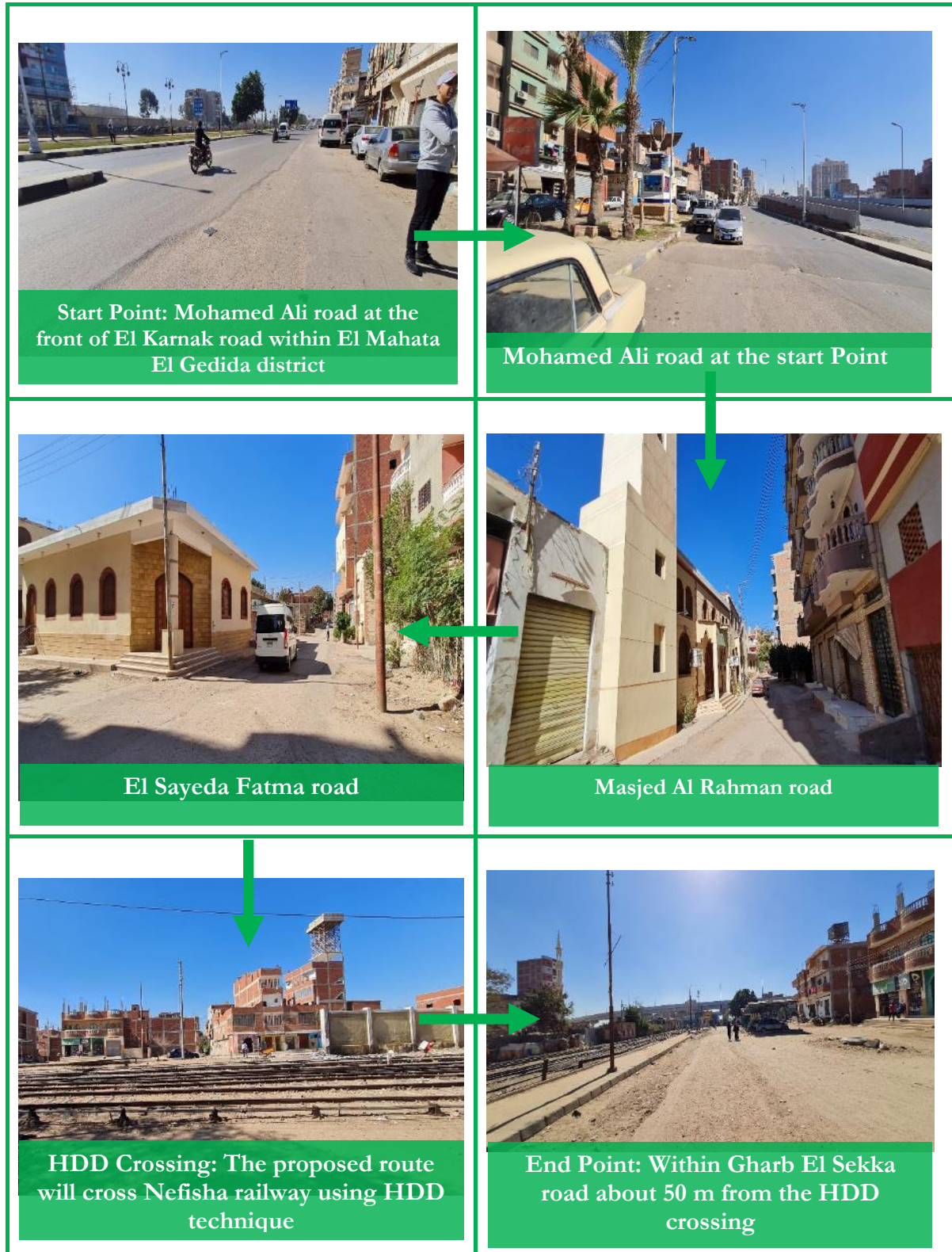
Figure 2-3: Pictures showing Nefisha intermediate pressure pipeline route.
