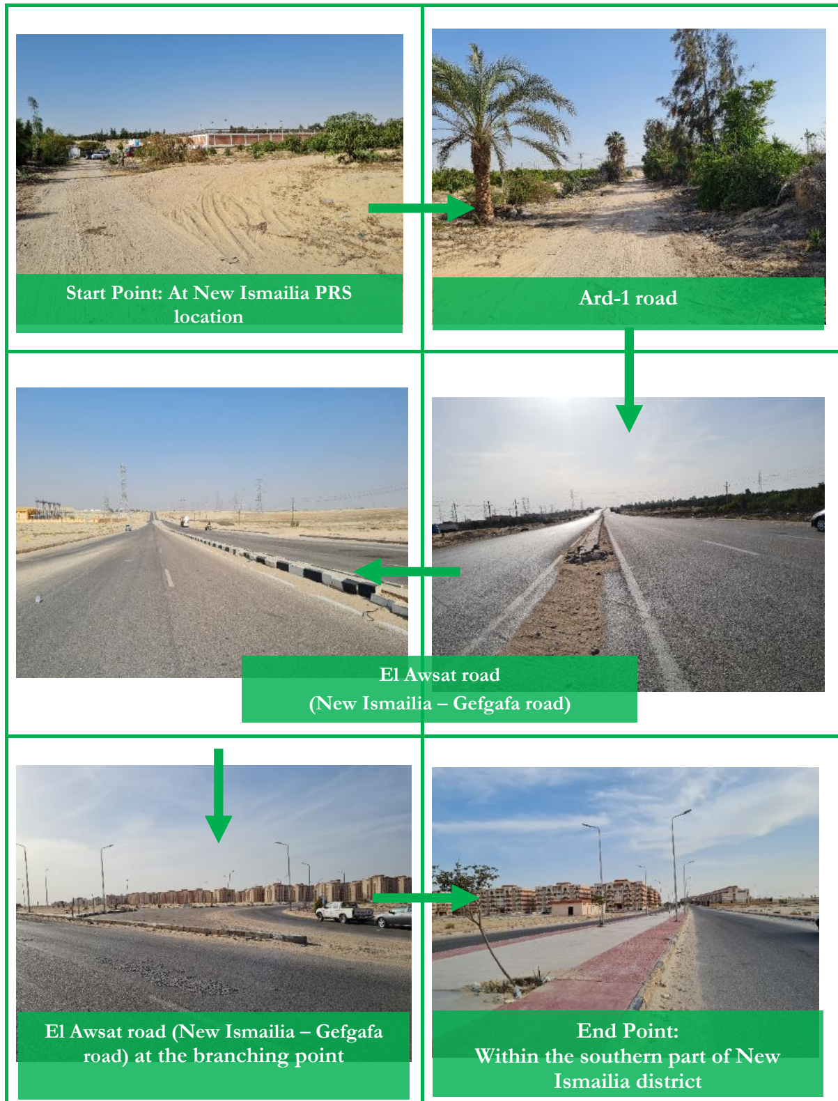
Figure 2-7: Pictures showing New Ismailia intermediate pressure pipeline route.
