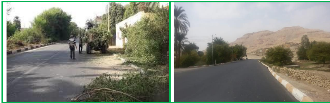
Figure 4-7: Pictures showing Streets Conditions at El Qarna.
