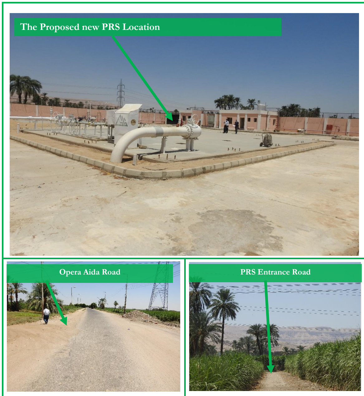
Figure 2-5: Pictures showing the proposed PRS and its surroundings
