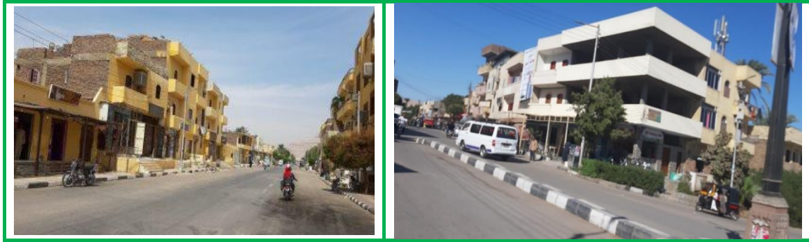
Figure 4-6: Pictures showing Building conditions at Markaz El Qarna.
