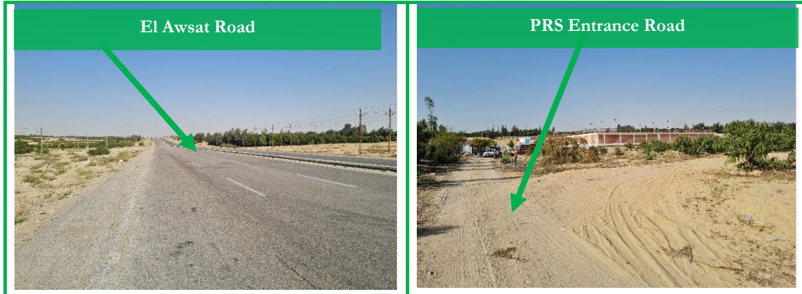
Figure 4-5: Shows the main roads closest to the new PRS area
