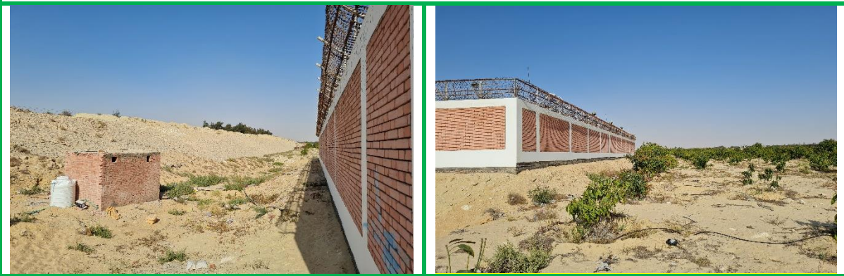
Figure 4-4: Shows Overview outside the proposed location for the new PRS
