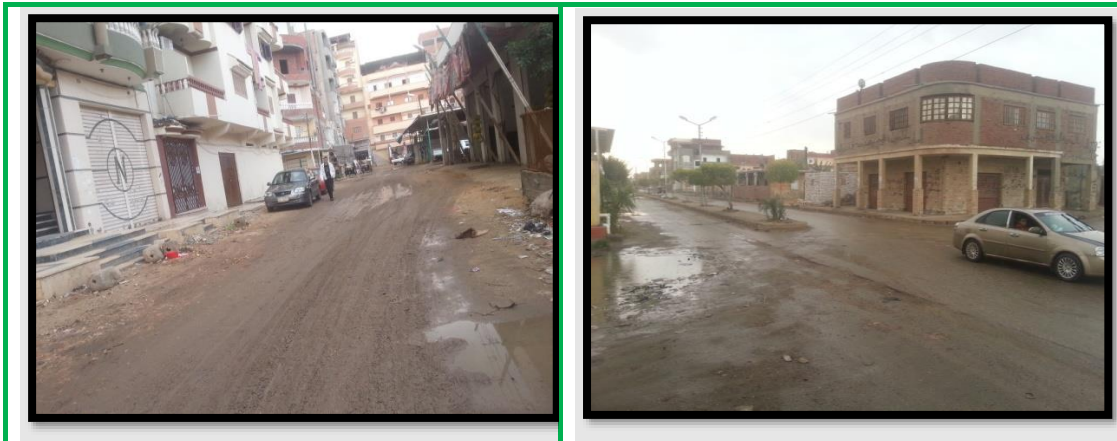
Figure 4-6: Pictures showing Building conditions at El Qantara East.
