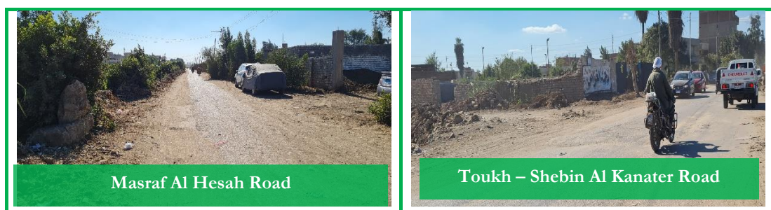
Figure 4-5: Shows the main roads closest to the new PRS area
