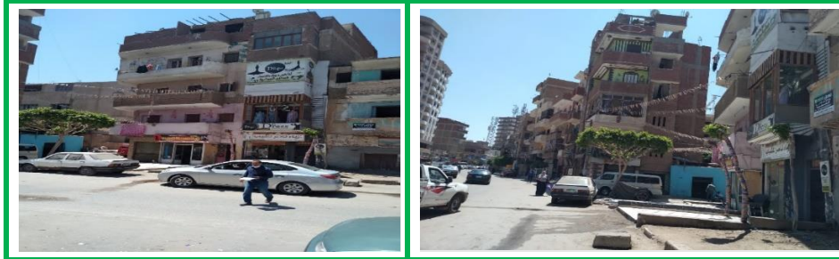
Figure 4-6: Pictures showing Building conditions at Markaz Toukh.
