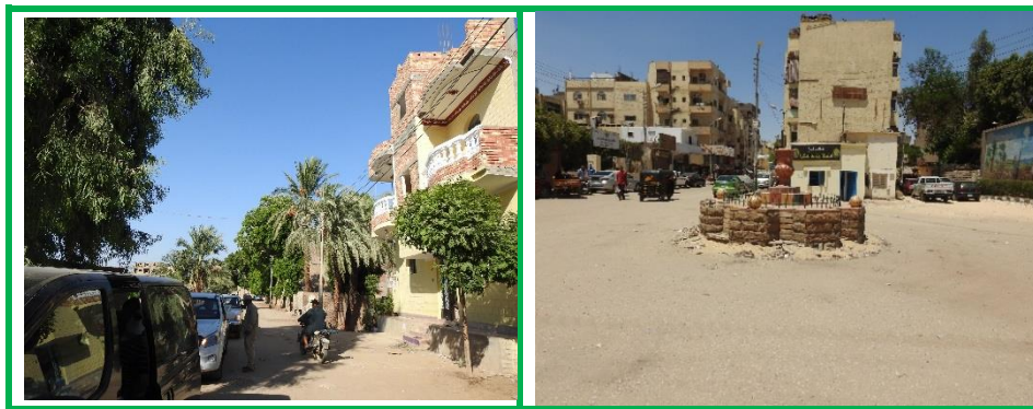
Figure 4-5: Pictures showing Building conditions at Markaz Armant.
