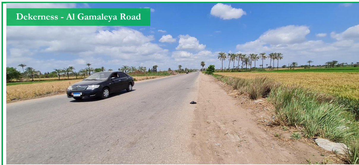
Figure 4-4: Shows the main road closest to the PRS area
