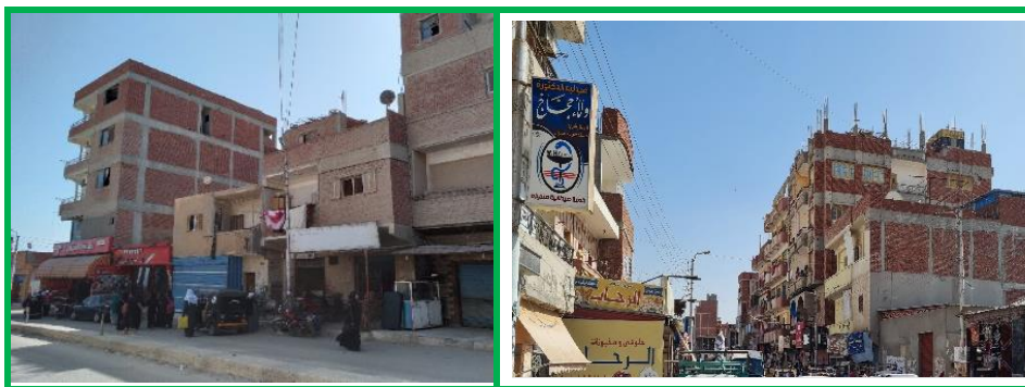
Figure 4-5: Pictures showing Building conditions at Markaz Dekerness.
