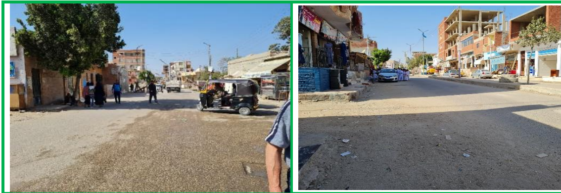
Figure 4-6: Pictures showing Streets Conditions at Markaz Dekerness.
