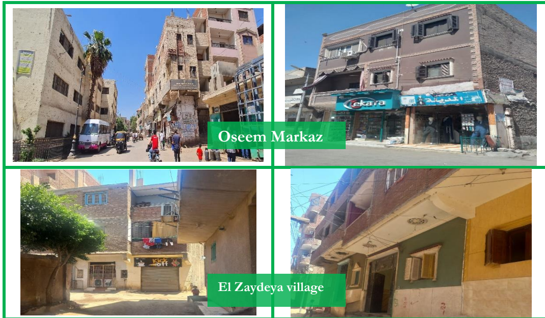
Figure 4-5: Pictures showing Building conditions at Markaz Oseem areas.
