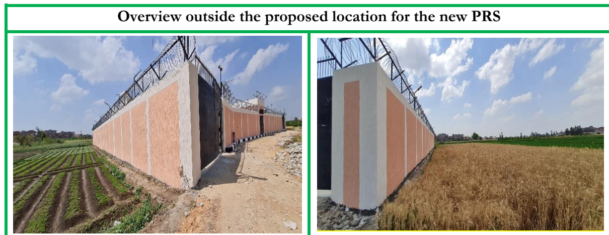
Figure 4-4: Shows Overview outside the proposed location for the new PRS
