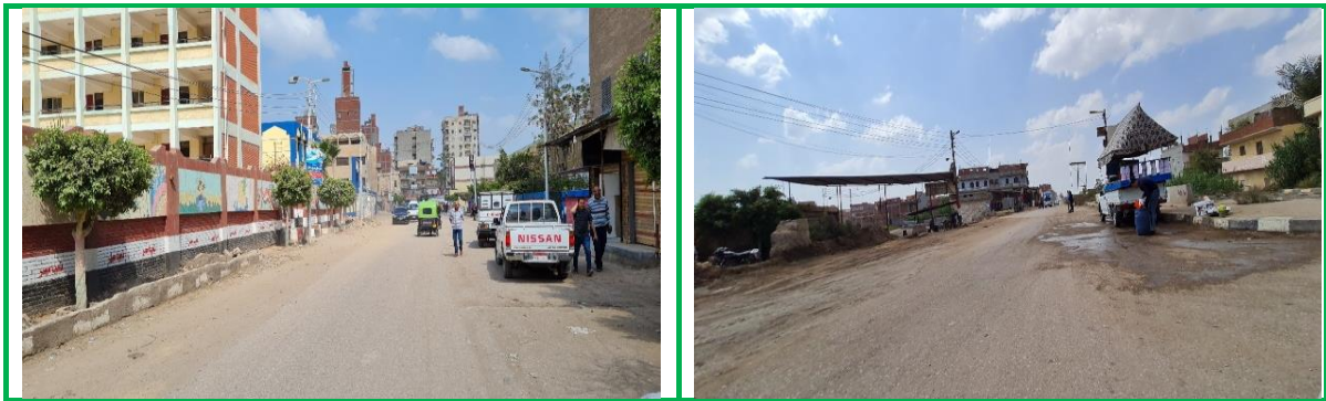
Figure 4-7: Pictures showing Streets Conditions at Markaz Qtor.
