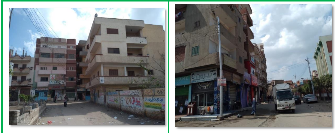
Figure 4-6: Pictures showing Building conditions at Qtor.
